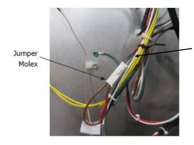
Cut the Molex plug and wire Zone 2 circulator to the remaining wires
